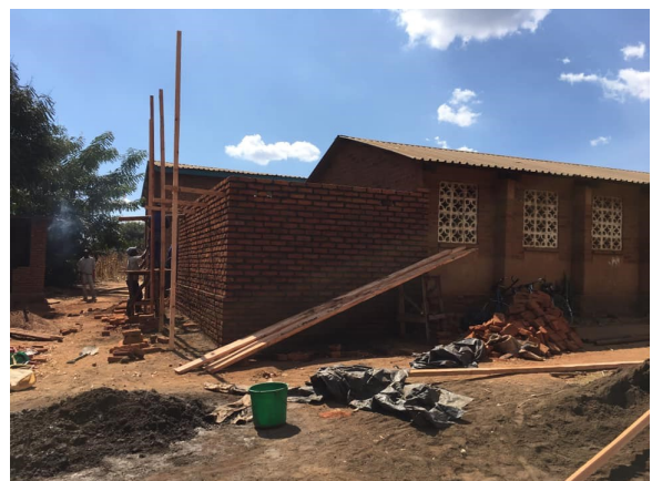
(Mwalaulomwe clinic renovations)
